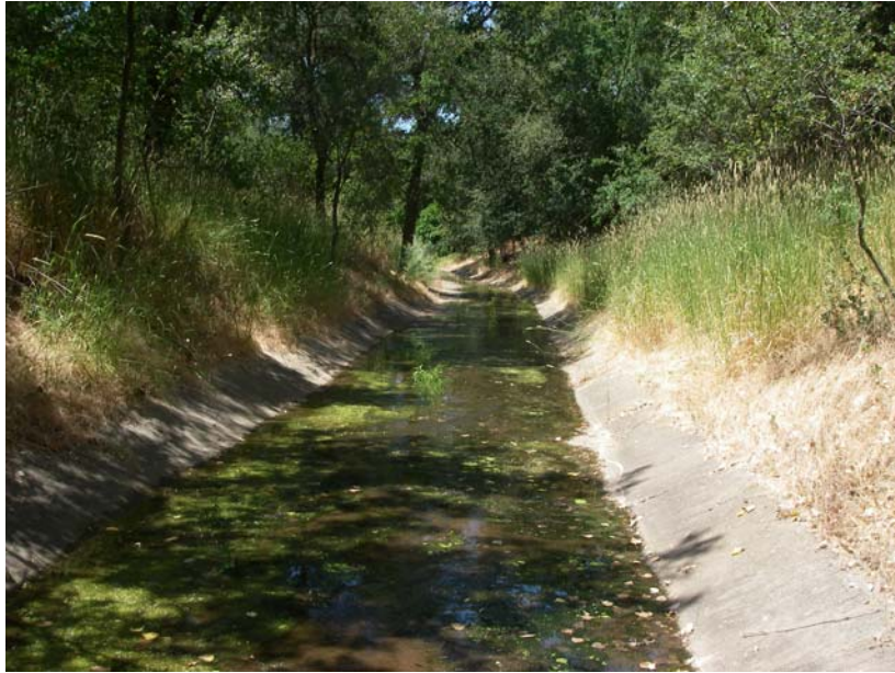
Concrete-Lined Channel (Reach 19)
