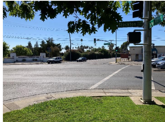
Figure 34. Large Curb Radii at Intersection of Stockton Boulevard and Lemon Hill Avenue
