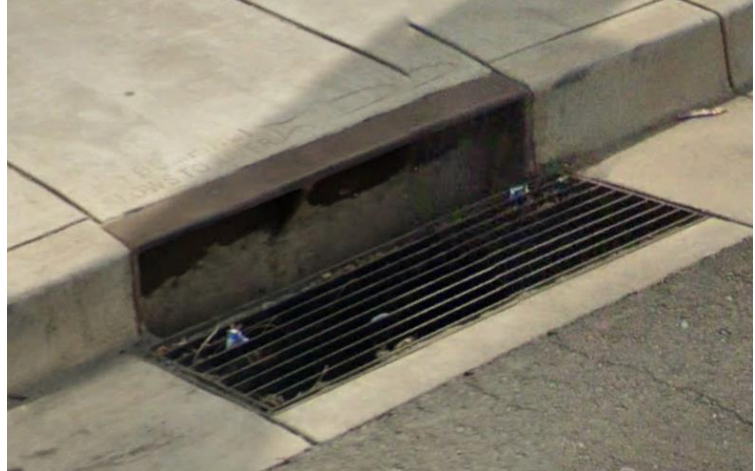
Figure 15. Parallel Drainage Grate along Norwood Avenue Bike Lane
