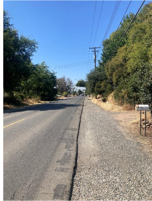
Figure 8. Missing Sidewalk along Marysville Road
