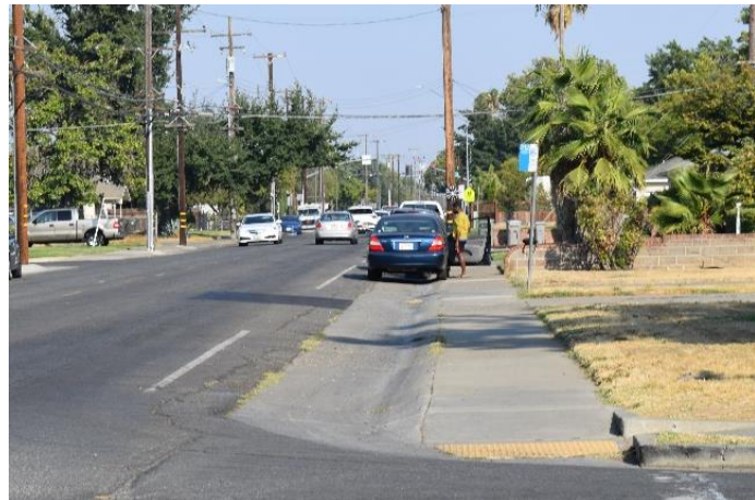
Figure 21. Rolled Curbs on 14th Avenue
