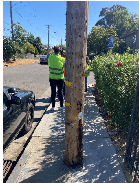
Figure 29. Utility Pole Obstructing Sidewalk on 63rd Street
