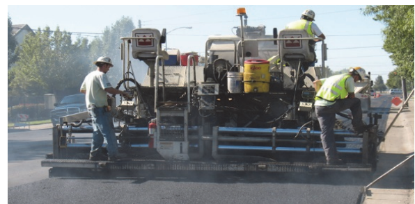
Street overlay in progress
