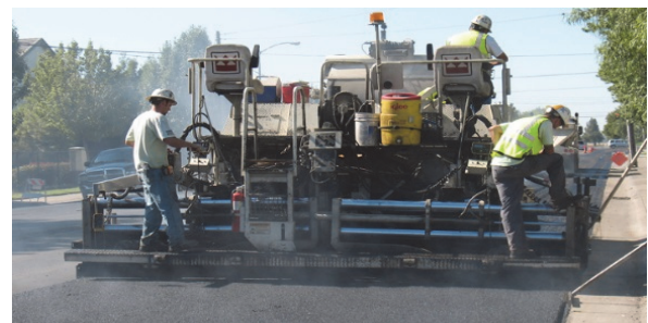
Street overlay in progress
