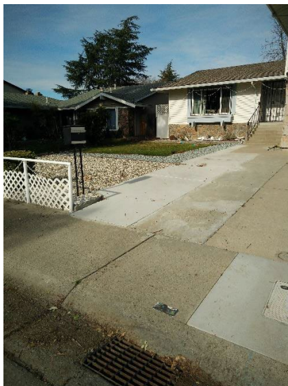
FIGURE 38. ELEVATED HOME WITH LANDSCAPING ASSISTING IN ON-SITE DRAINAGE
