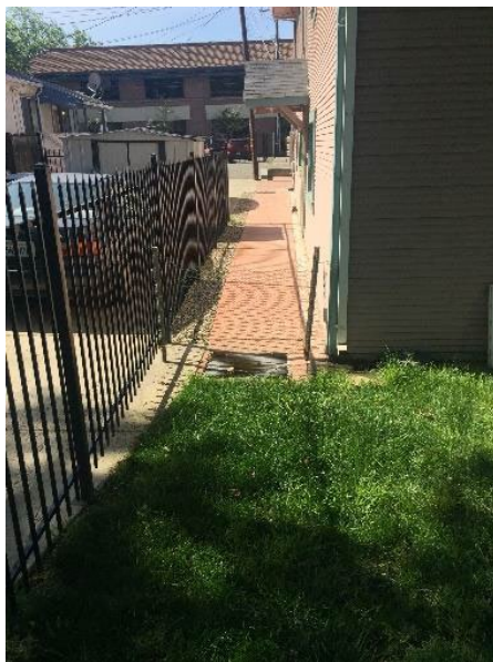
FIGURE 17. ON-SITE DRAINAGE ADDED TO AID IN STORMWATER DRAINAGE
