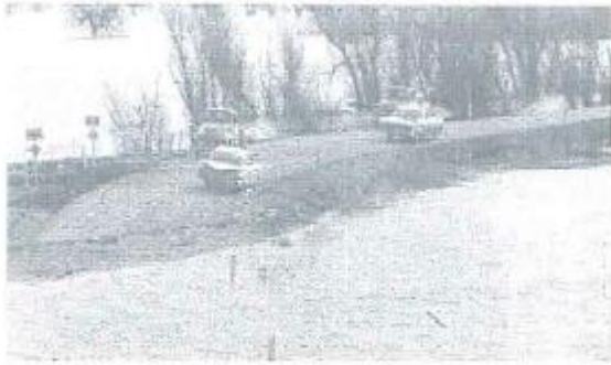
Figure 2.14. Flooding on Franklin Boulevard in 1964
