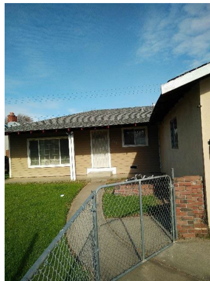
FIGURE 39. ELEVATED STRUCTURE WITH A CRAWL SPACE BELOW AS A FLOOD PROTECTION METHOD
