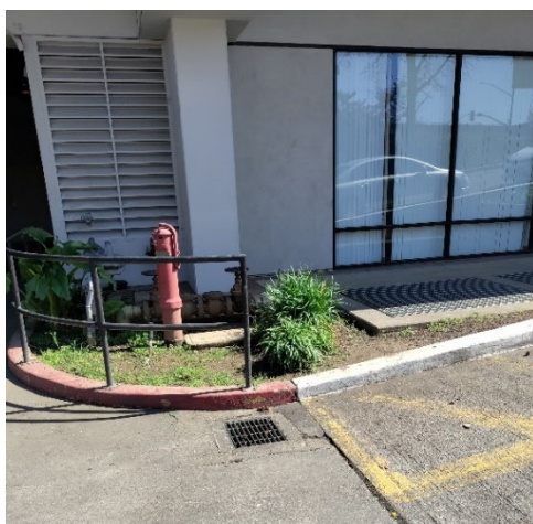
FIGURE 25. CURB AND GUTTER AT BASE OF RAMP TO STREET ABOVE
