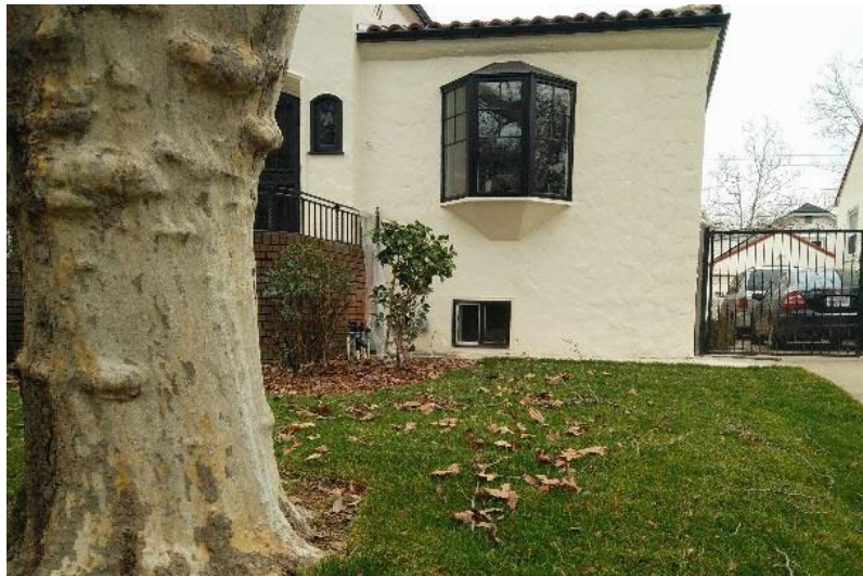
FIGURE 15. SOME HOMES IN THIS AREA HAVE BASEMENTS AND DOORWAYS LOCATED AT GRADE LEVEL
