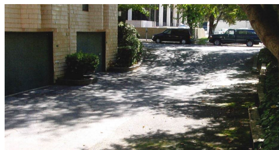
FIGURE 23. GARAGES ARE LOCATED BELOW GRADE.
