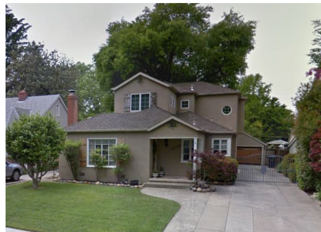
FIGURE 20. EXAMPLE OF A TYPICAL HOME IN THIS AREA THAT WOULDN'T FLOOD; ELEVATED ON A CRAWL SPACE AND THE GARAGE LOCATED IN THE BACK OF THE PROPERTY. SOME HOMES HAVE BASEMENTS
