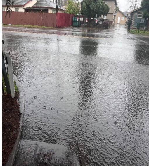
FIGURE 44. CLOGGED DRAINAGE INLET ON PALMER ST AND ARCADE BLVD
