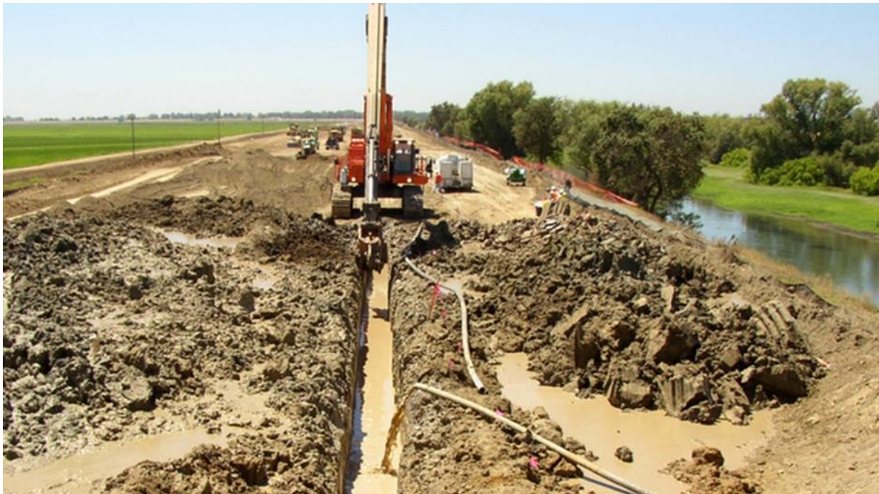
Figure 5.4. Natomas Levee Slurry Wall Construction
