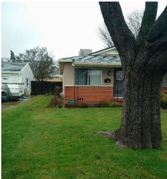
FIGURE 30. STRUCTURE BUILT ON A CRAWL SPACE AND HVAC UNIT IS ELEVATED AS A FLOOD-PROOFING MEASURE
