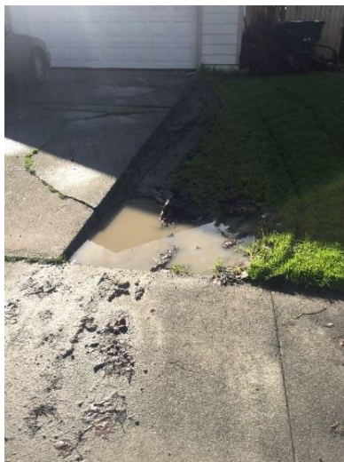
FIGURE 40. EXAMPLE OF FLOODED YARD FROM JANUARY 2017 STORMS
