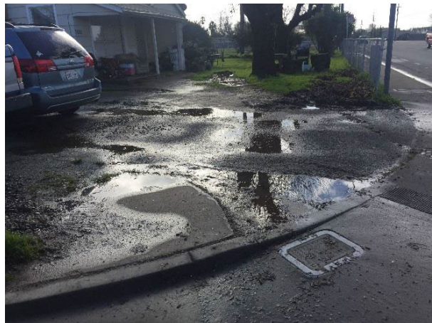
FIGURE 34. FRONT YARDS INUNDATED BY STREET FLOODING; PICTURES TAKEN TWO DAYS AFTER A LARGE STORM
