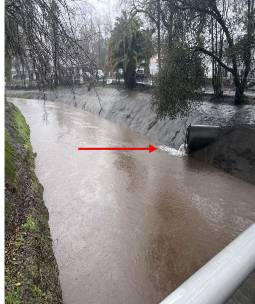
FIGURE 46. ARCADE CREEK LOOKING WEST FROM VERANO BRIDGE (STAGE 40-42 FT AT MARYSVILLE BLVD (CITY) (47403); JANUARY 5
