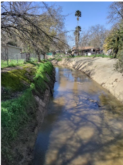
FIGURE 47. ARCADE CREEK LOOKING WEST FROM VERANO BRIDGE
