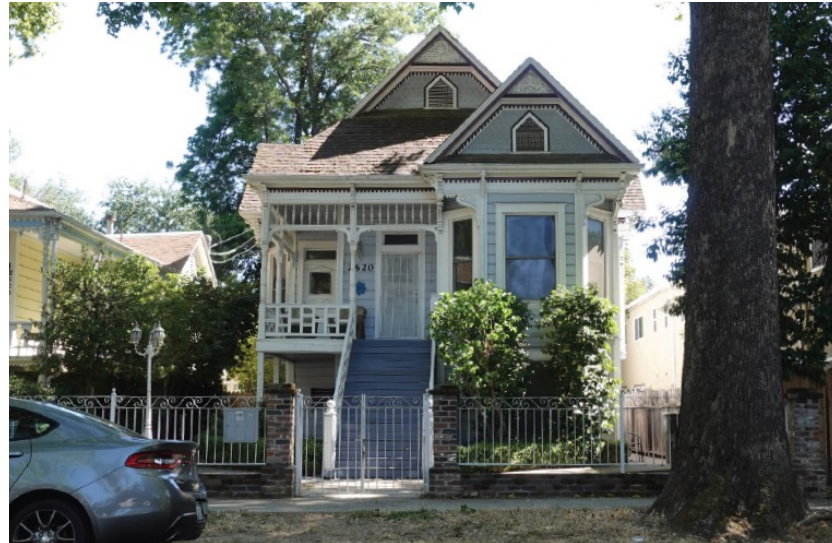
Tier 2 District (4+2) (31% of City's residential land) 4 Primary Units + 2 ADUs Typical MMH: Fourplex
