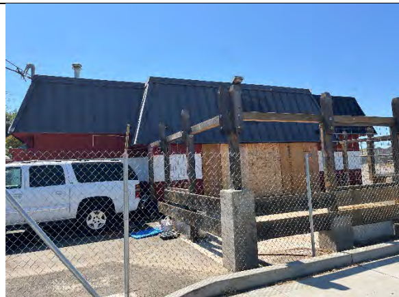
Figure 1. North facade, view southwest.
