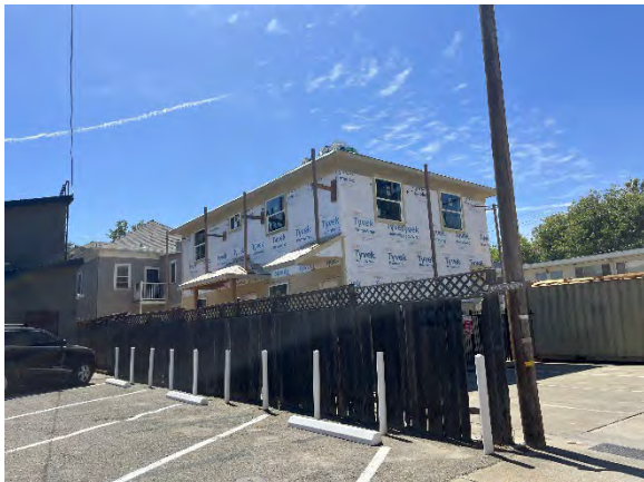
Figure 3. Partial view of the rear façade and detached ADU, view southwest.
