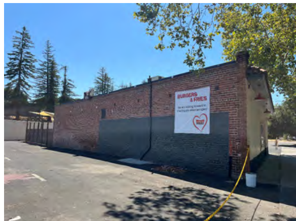
Figure 3. North facade, view southeast.
