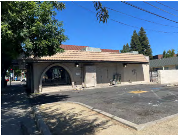
Figure 3. Southwest facade, view north.
