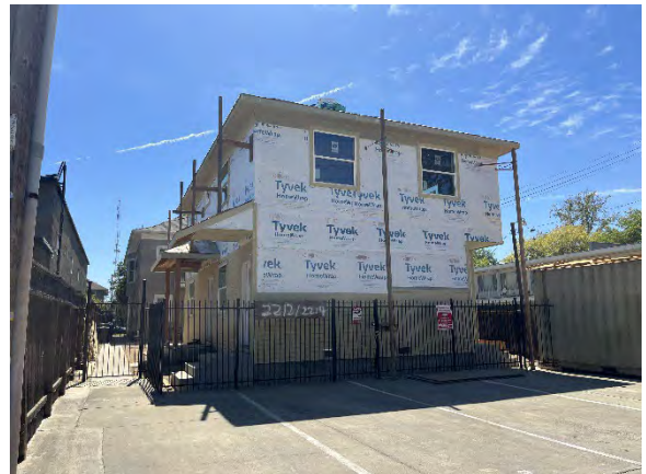
Figure 4. Context view of detached ADU, view southwest.
