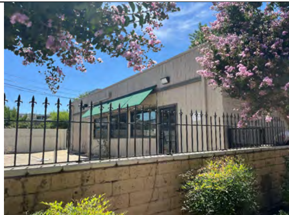
Figure 4. Southeast façade, view west.
