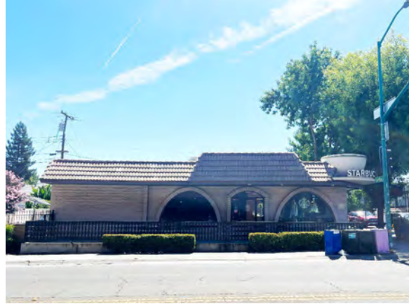
Figure 2. Northeast facade, view southeast.
