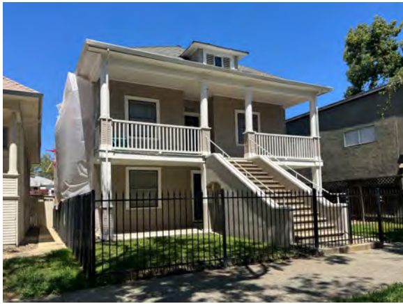
Figure 1. Primary south facade, view northeast.
