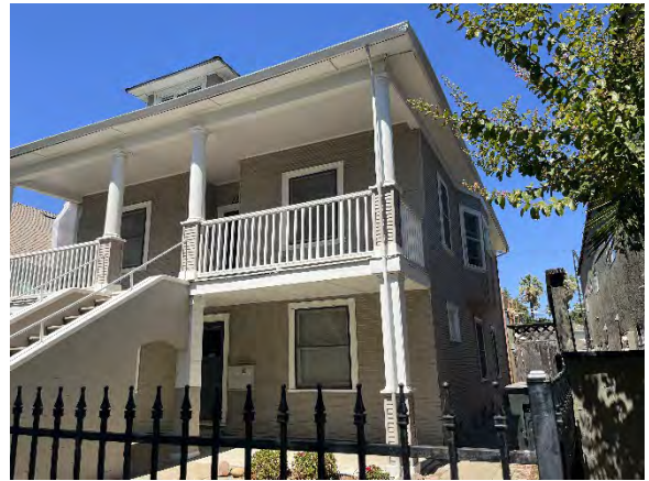
Figure 2. Oblique view of south and east facades, view north.
