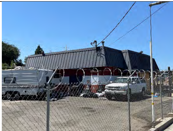
Figure 2. East facade, view southwest.
