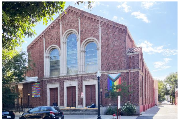
2100 J Street (APN 007-0091-001-0000) First United Methodist Church. The church hosted meetings for early homophile groups in the late 1960s and has continuously welcomed members of the
