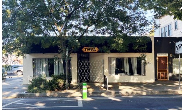
910-912 21st Street (APN 007-0016-010-0000) Offices of Dr. Harvey Thompson and Dr. Sandy Pomerantz and the Open Book bookstore. The building housed the medical offices of Dr. Thompson and Dr. Pomerantz from 1978-1987 and the Open Book from 1996 to 2005.
