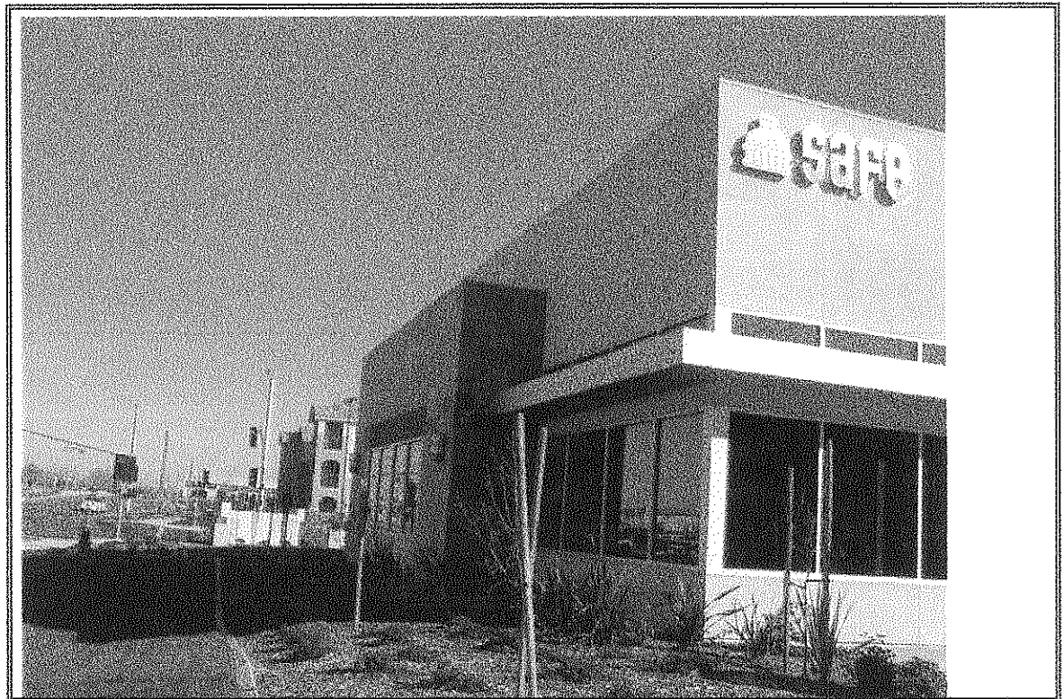
Photograph Number 6 West side of 2200 Building
