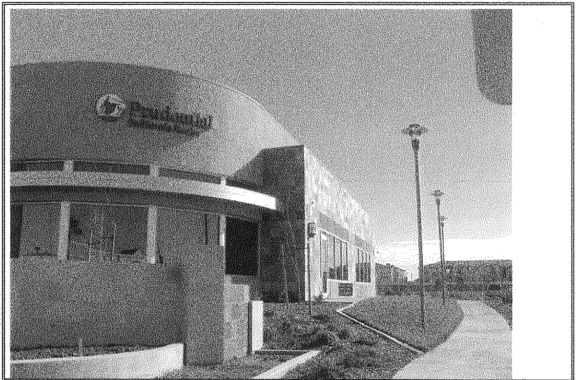
Photograph Number 10: West side of 2250 Building
