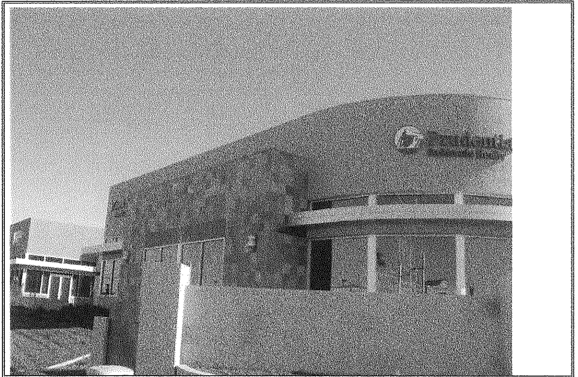
Photograph Number 9: Northwest side of 2250 Building
