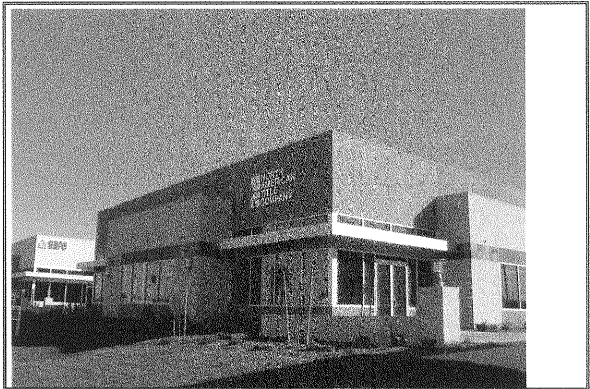
Photograph Number 8 Northwest side of 2230 Building
