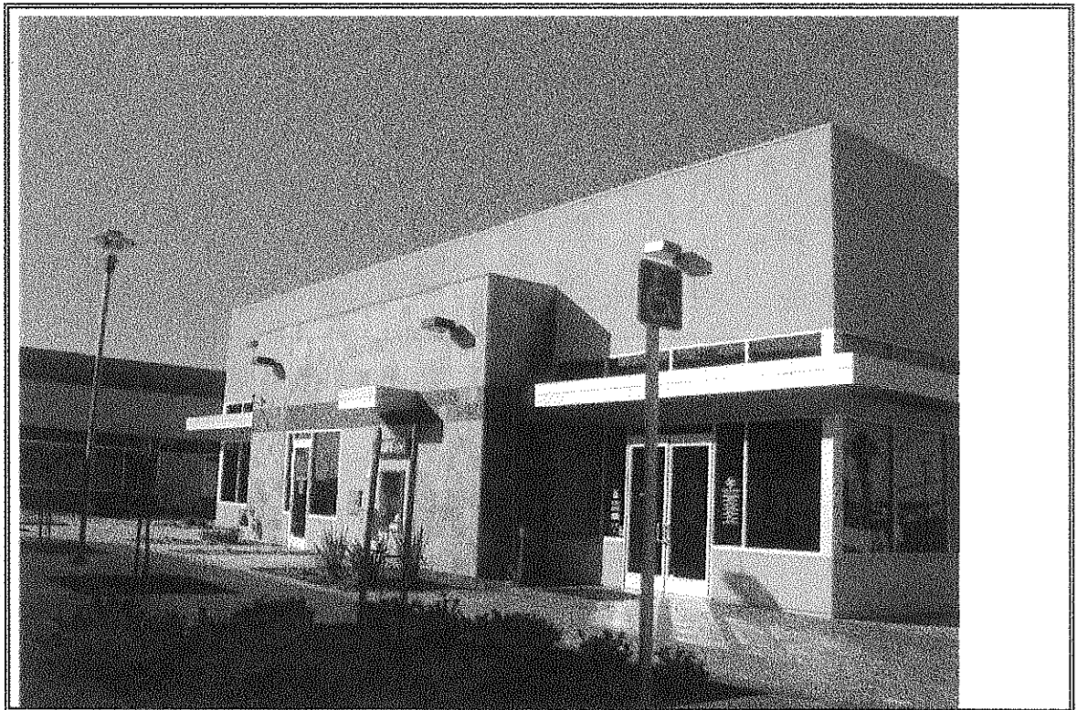
Photograph Number 16 South side of 2200 Building
