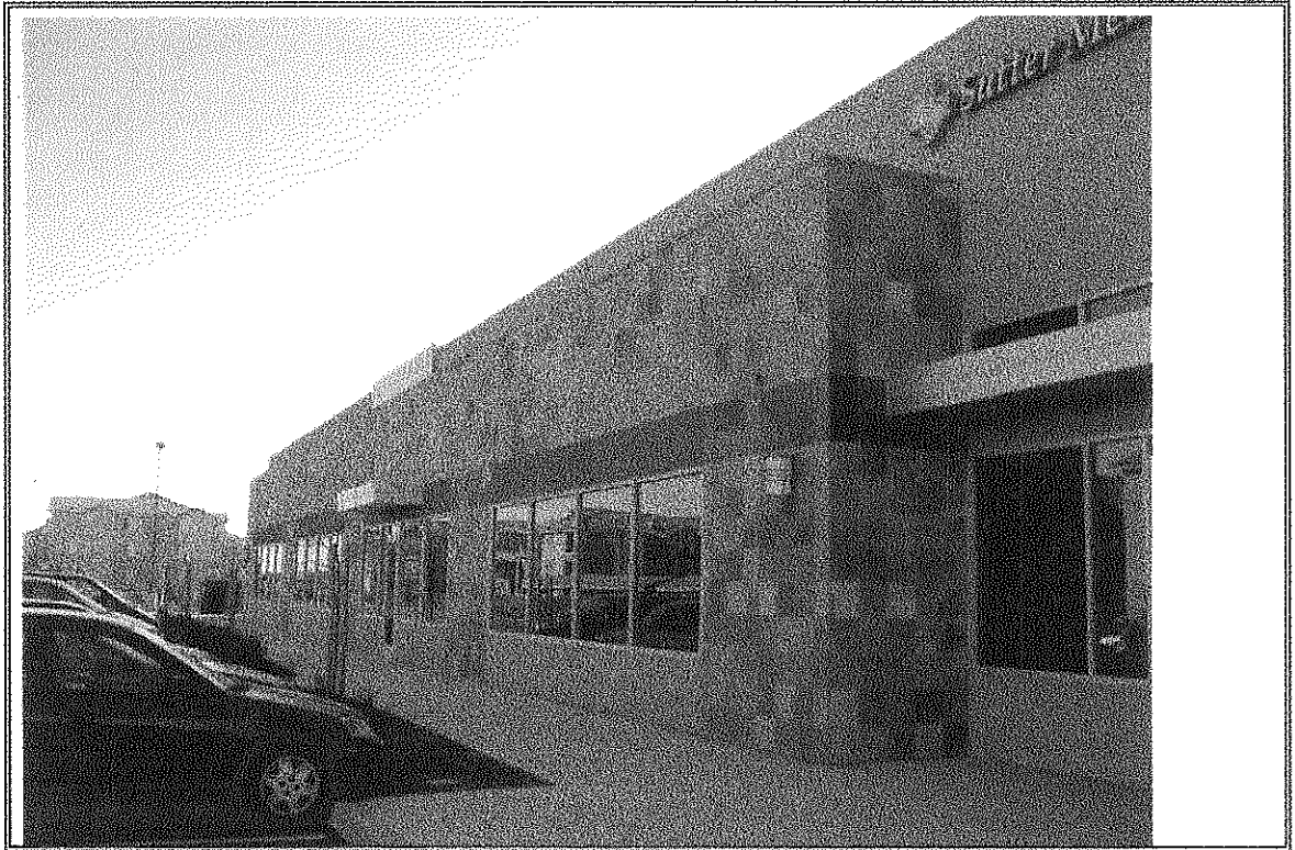
Photograph Number 15: East side of 2210 Building
