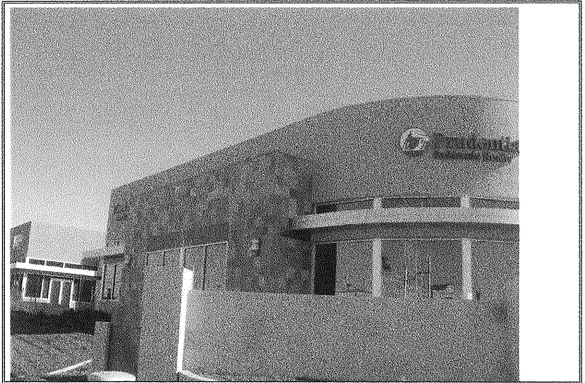
Photograph Number 9: Northwest side of 2250 Building
