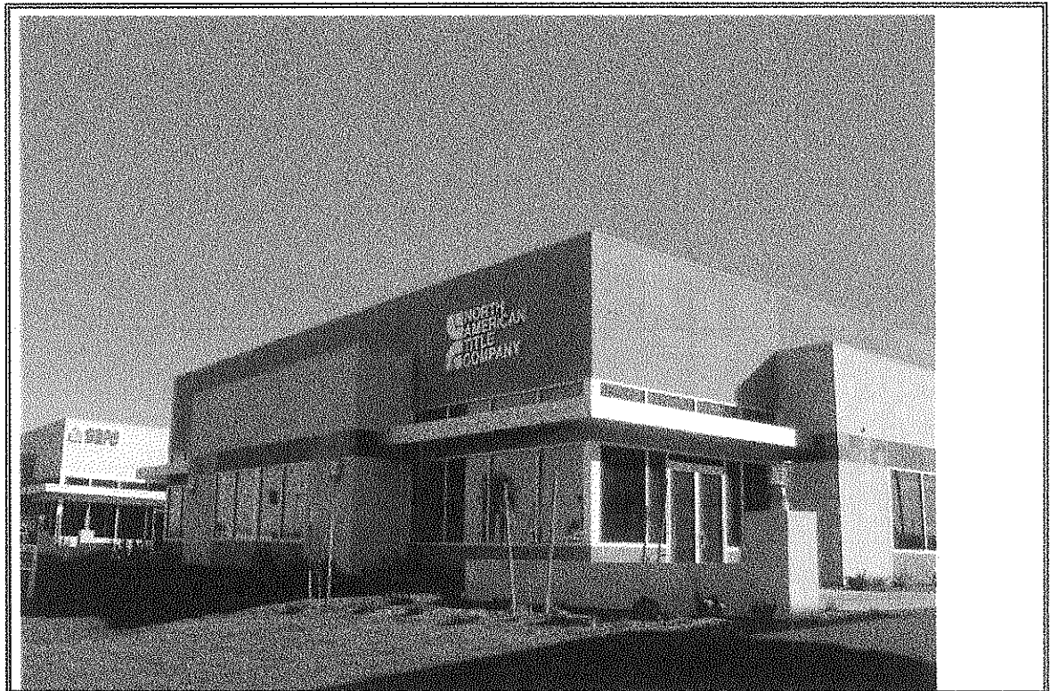
Photograph Number 8 Northwest side of 2230 Building
