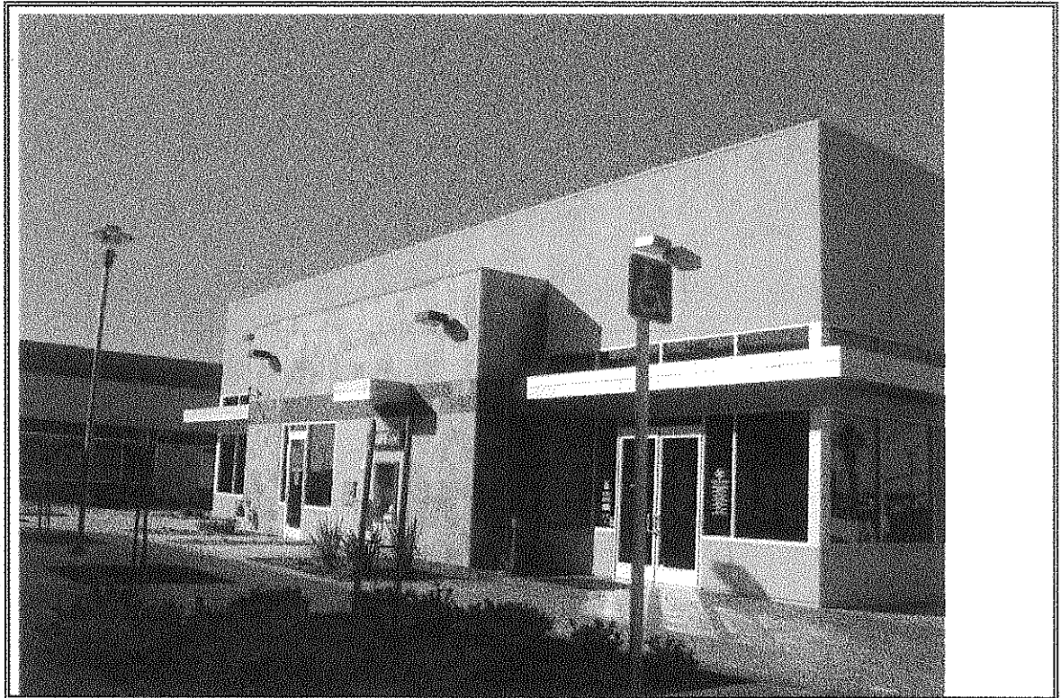
Photograph Number 16 South side of 2200 Building
