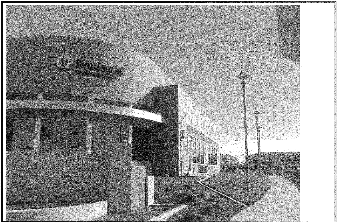
Photograph Number 10: West side of 2250 Building
