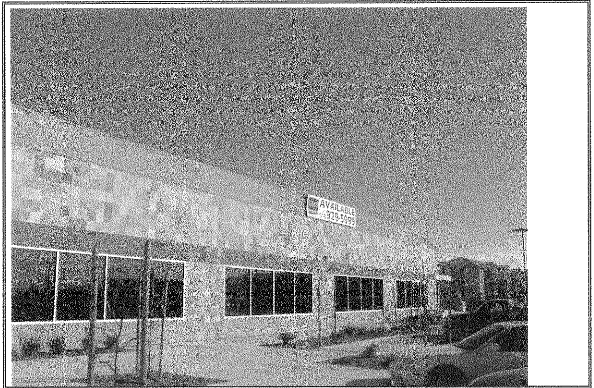
Photograph Number 5: West side of 2210 Building
