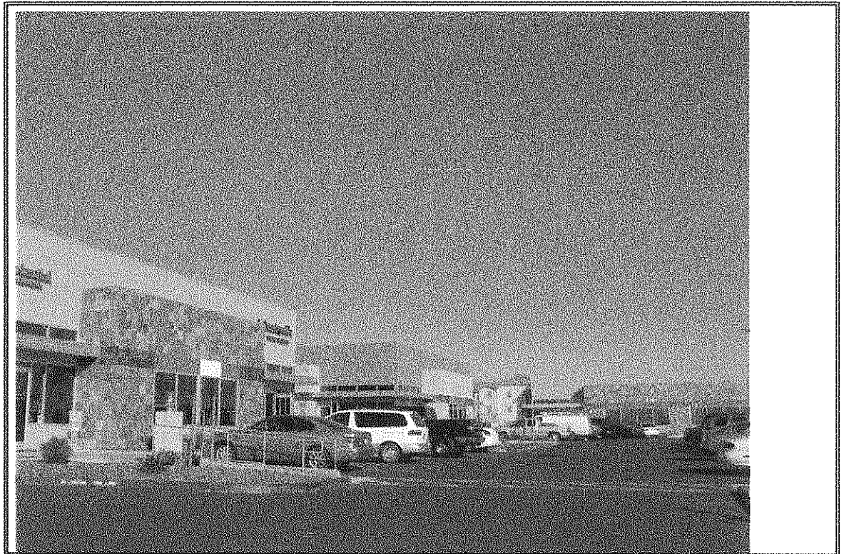
Photograph Number 12 South side of 2250 and 2230 Buildings, parking area and west side of 2210 Building
