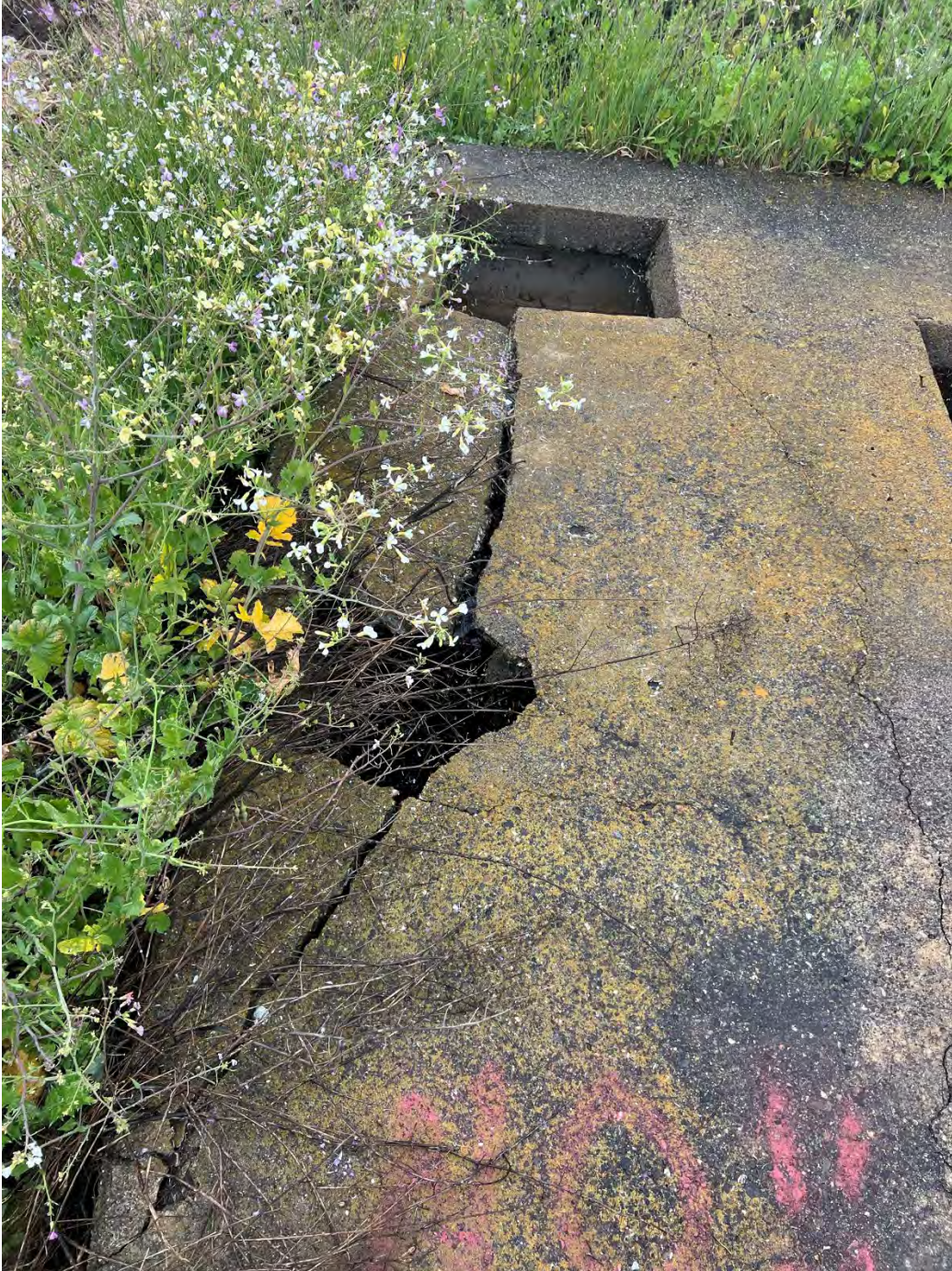
Photo 3 RBTS 002 Facing West
