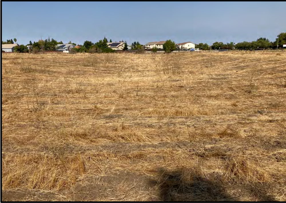
Slightly low area in the south part of the site, looking north from the south edge of the site; 10/18/23. The site was graded in 2007/2008 for an office complex (that was not built), leaving a few low areas and three slightly elevated pads in the site.
