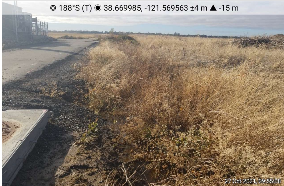
Photo 1. The north end of Ditch-1, looking south from Bayou Way.
