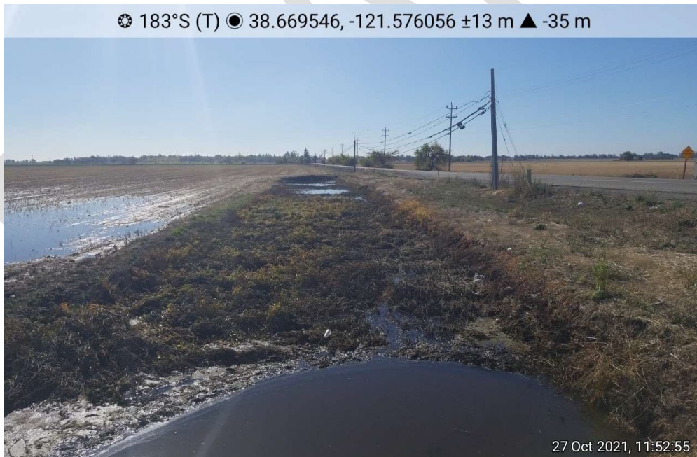
Photo 4. Canal-1 along Powerline Road, looking south towards OHWM SP-3. A significant rain event occurred prior to conducting the survey, causing the canal to flood and an excess of stormwater sheet flow to pond in the adjacent agricultural field.
