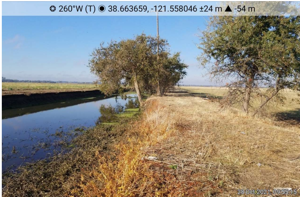
Photo 7. Canal-3 (West Drainage Canal), looking west towards OHWM SP-5, located just west of where Canal-2 discharges to Canal-3.
