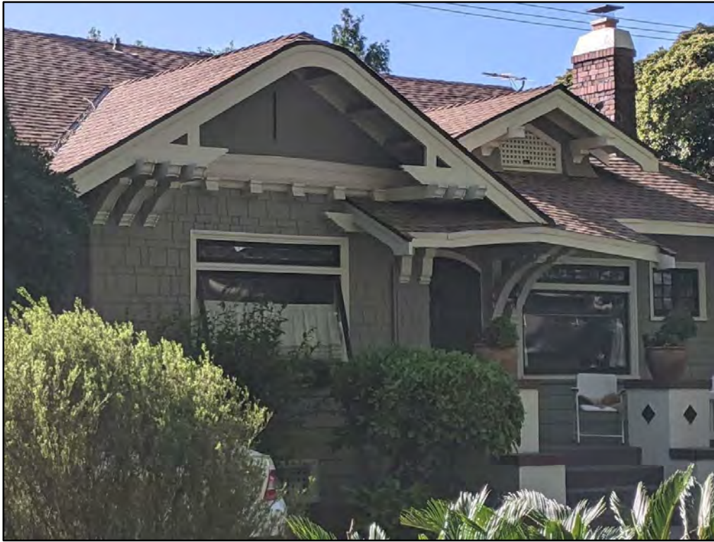
Detail view of Craftsman features on south end of façade.
