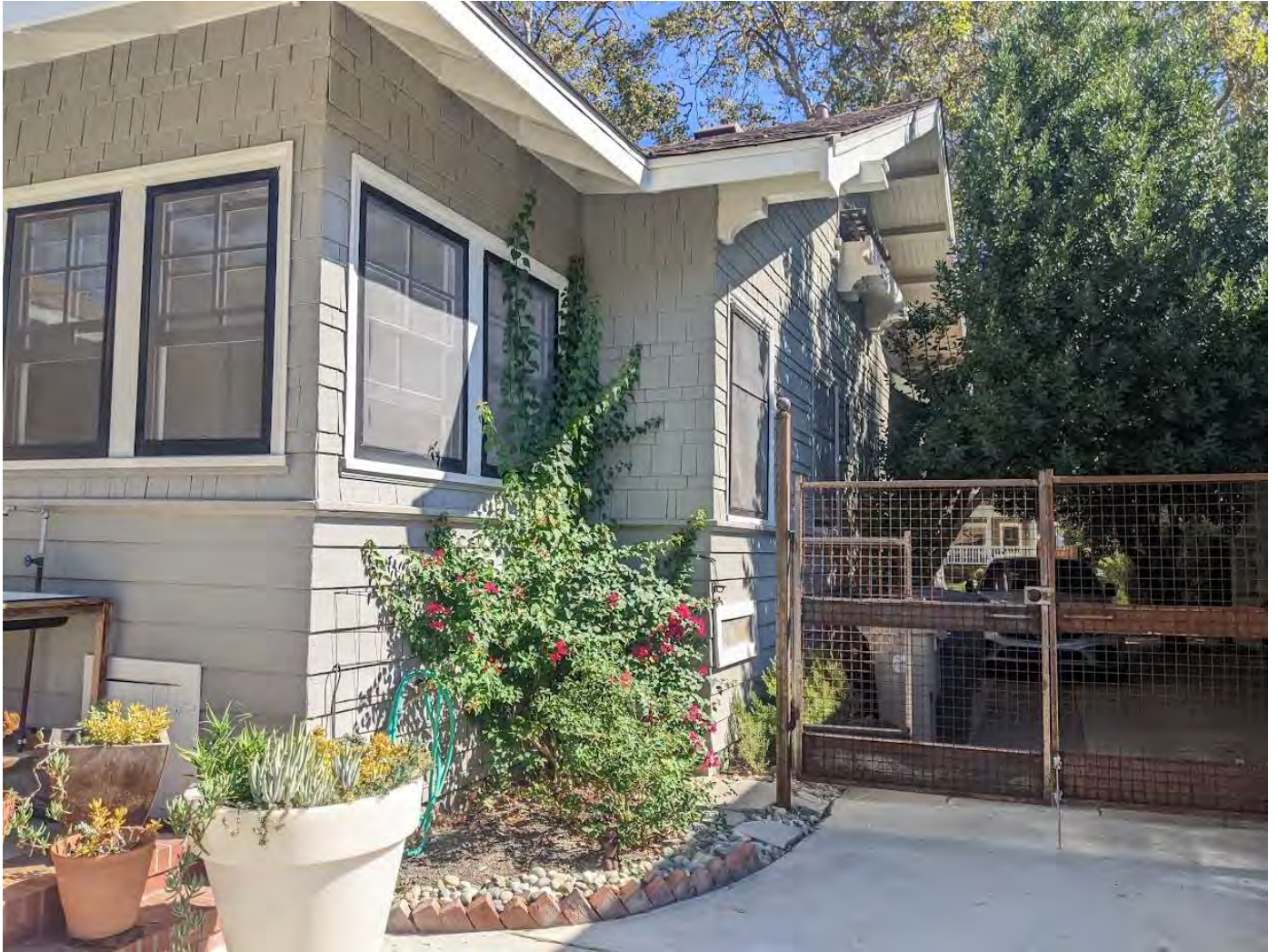
South West Elevation (Partial South Side) Detailed window box from the attic.
